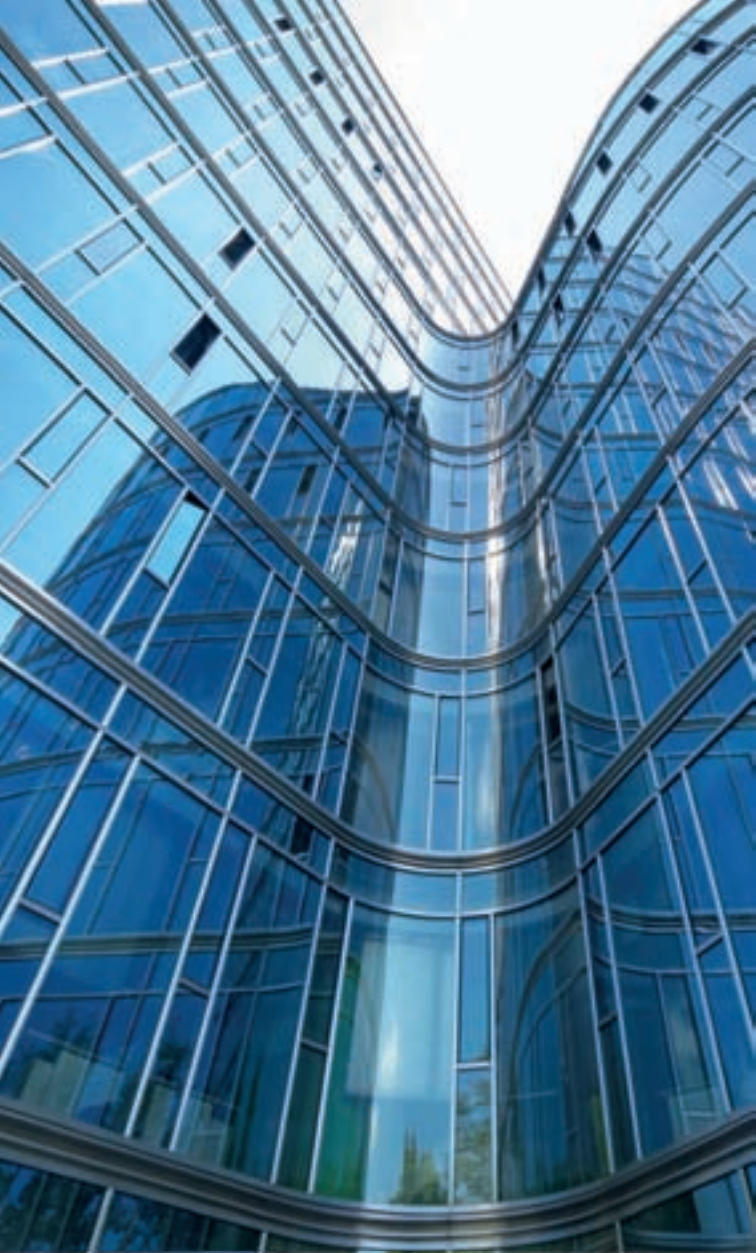
Ambassador Office Building – Warszawa, Polska – Architekt: AMC – Andrzej M. Choldzynski Sp. z o. o. – Stopray Vision-50 +
