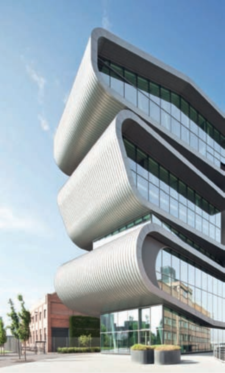
Umicore – Hoboken, Belgia – Architekt: Conix Architects – Thermobel Stopray Vision-50 i Vision-50 T
