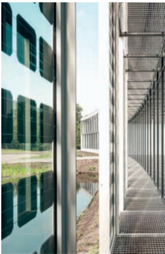
AGC Technovation Center – Gosselies, Belgia – Architekt: ASSAR Architects – SunEwat XL
