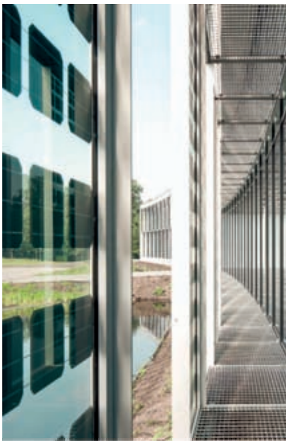
AGC Technovation Center – Gosselies, Belgie – Architekt: ASSAR Architects – SunEwat XL
