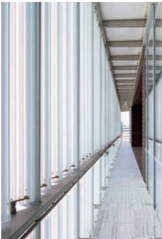
AGC Glass Building – Louvain-la-Neuve, Belgie – Architekt: Philippe Samyn and Partners – Sklenné žaluzie z vrstveného skla s potiskem Planibel Clearvision © AGC Glass Europe – Philippe SAMYN and PARTNERS sprl, architects and engineers – BEAI sa
