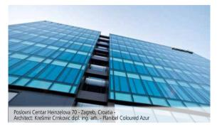
The Planibel Coloured range comprises body tinted glass which can be used for solar control applications.
