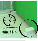
In moist areas, always seal joints. Whilst sealing joints, protect glass with masking tape and remove tape as soon as silicone is applied.
