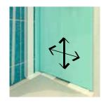
Once well positioned, press firmly on glass for adhesion to tape.
