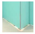
Allow at least 48h drying time before removing setting blocks.
