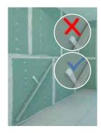
Apply FIX-IN PR wall primer on porous surfaces and let it dry. Some Lacobel, Imagin Backpainted and Matelac colours require a uniform painted background (see p. 3). No wall primer needed in case of white painted background.
