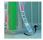
Start installation at outer edge. Position and adjust the sheet whilst floating on silicone.
