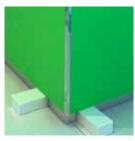
Allow at least 48h drying time before removing setting blocks.
