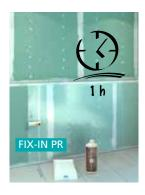
Paint a narrow line (max 1cm) on the joint areas in colours matching the glass and let it dry.
