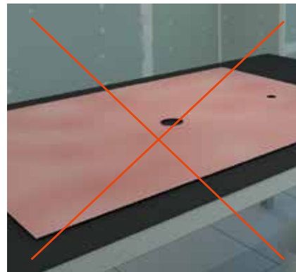
WRONG: NO SURFACE ACTIVATOR SILICONE
