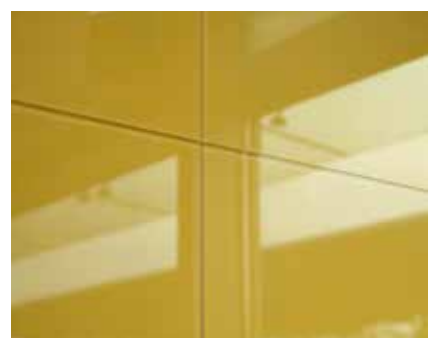
JOINTS WITH SILICONE
