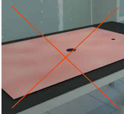
WRONG: NO SURFACE ACTIVATOR SILICONE
