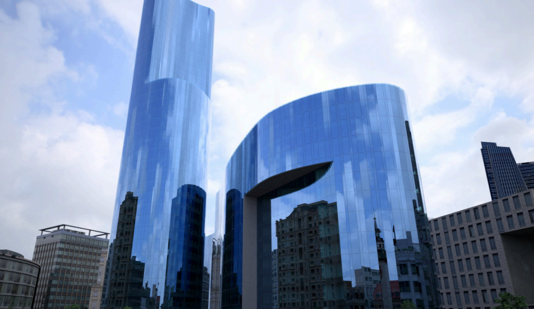
Stopray Blue Ace-30T 6mm - 16mm 100% Air - Clear float 6mm, cloudy environment
