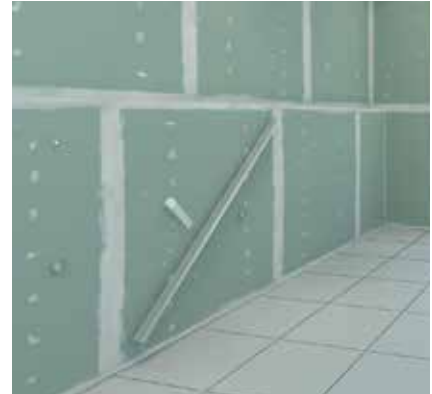
MEASUREMENT OF FLATNESS OF THE WALL
