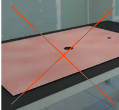
WRONG: NO SURFACE ACTIVATOR SILICONE
